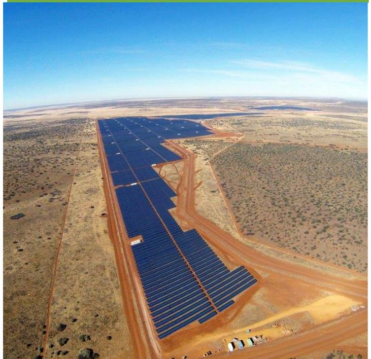
The Jasper solar farm, located near Kimberley in South Africa, is now the continent's largest solar power project. Construction was completed in October 2014, and it is now fully operational. With a rated capacity of 96 megawatts, Jasper will produce about 180,000 megawatt-hours of clean energy annually for South African residents, enough to power up to 80,000 homes.
